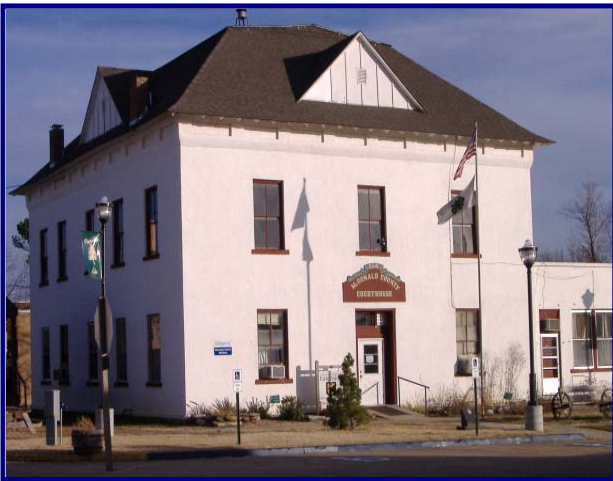
Old Courthouse, Pineville, Missouri – 2006
